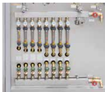
Cooling water distribution
